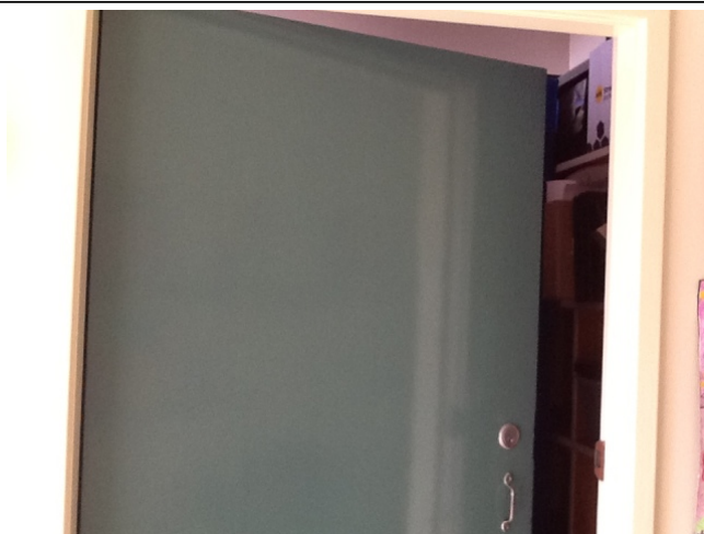
Photo No: J128920-003-Photo008 Result: Lead (Paint) - Presumed Positive Building/Level: Building A-Ground Level Room/Location: R0003-North Feature/Material: Door-Paint System/s
