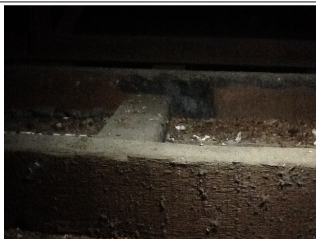
Photo No: J128920-003-Photo031 Result: Lead (Dust) - Positive Building/Level: Building A-Ground Level Room/Location: Ceiling Space-North Feature/Material: On Top of Ceiling-Dust - Lead
