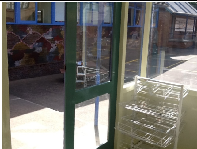
Photo No: J128920-003-Photo004 Result: Lead (Paint) - Positive Building/Level: Building A-Ground Level Room/Location: R0002-Throughout Feature/Material: Door-Paint System/s
