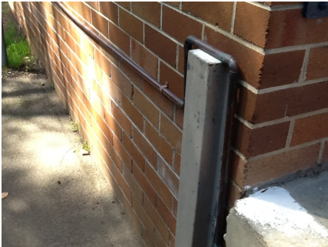
Photo No: J128920-003-Photo058 Result: Lead (Paint) - Positive Building/Level: Building C-Ground Level Room/Location: Exterior-West Feature/Material: Metal Work-Paint System/s
