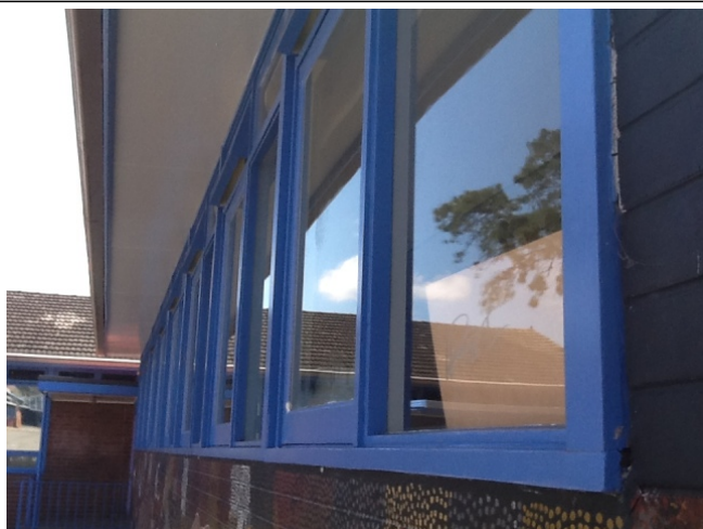
Photo No: J128920-003-Photo041 Result: Lead (Paint) - Positive Building/Level: Building A-Ground Level Room/Location: Exterior-North & West Feature/Material: Window Frame-Lower Paint System/s
