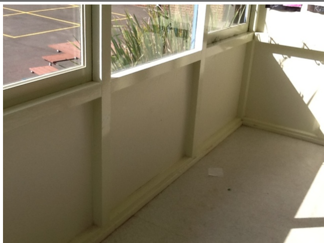
Photo No: J128920-003-Photo003 Result: Asbestos - Previously Sampled Positive Building/Level: Building A-Ground Level Room/Location: R0002-Throughout Feature/Material: Wall Lining-Fibre Cement Sheetting
