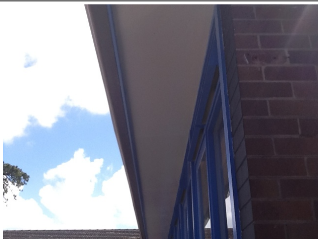
Photo No: J128920-003-Photo036 Result: Asbestos - Previously Sampled Positive Building/Level: Building A-Ground Level Room/Location: Exterior-Throughout Feature/Material: Eaves-Flat Cement Sheetting
