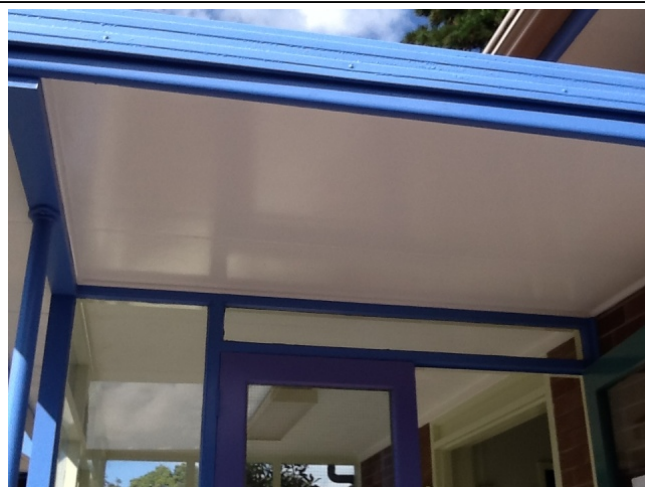
Photo No: J128920-003-Photo001 Result: Asbestos - Previously Sampled Positive Building/Level: Building A-Ground Level Room/Location: Movement - R0016-Throughout Feature/Material: Ceiling-Fibre Cement Sheet
