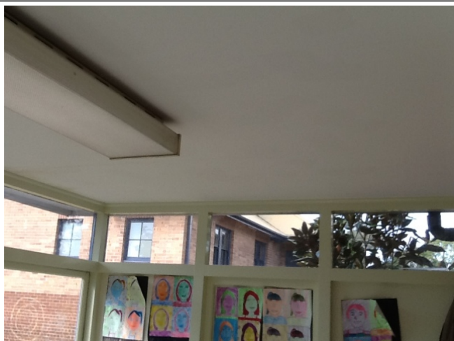
Photo No: J128920-003-Photo002 Result: Asbestos - Previously Sampled Positive Building/Level: Building A-Ground Level Room/Location: R0002-Throughout Feature/Material: Ceiling-Fibre Cement Sheetting
