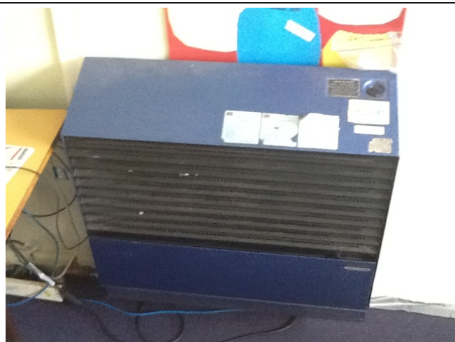
Photo No: J128920-003-Photo025 Result: Asbestos - Presumed Positive Building/Level: Building A-Ground Level Room/Location: R0010-South Feature/Material: Heater-Insulation
