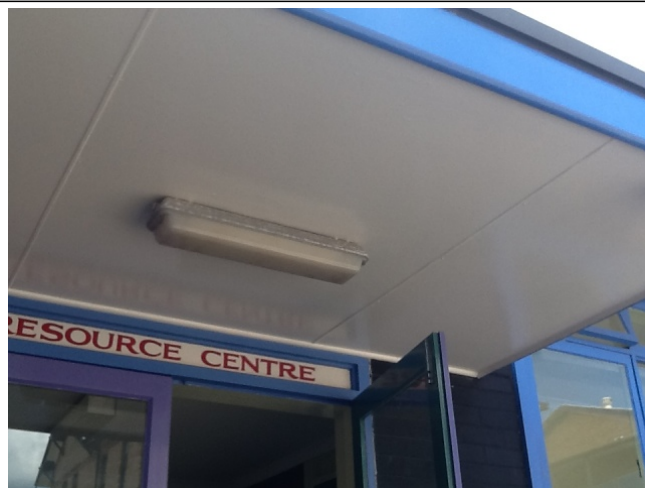
Photo No: J128920-003-Photo037 Result: Asbestos - Previously Sampled Positive Building/Level: Building A-Ground Level Room/Location: Exterior-Throughout Feature/Material: Awning-Flat Cement Sheetting
