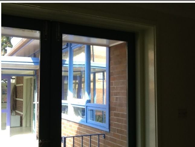
Photo No: J128920-003-Photo016 Result: Lead (Paint) - Presumed Positive Building/Level: Building A-Ground Level Room/Location: Movement - AR0019-North Feature/Material: Door-Paint System/s
