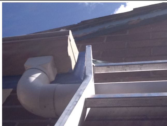
Photo No: J128920-003-Photo034 Result: Asbestos - Positive Building/Level: Building A-Ground Level Room/Location: Exterior-Throughout Feature/Material: Gable Verge Lining-Flat Cement Sheetting
