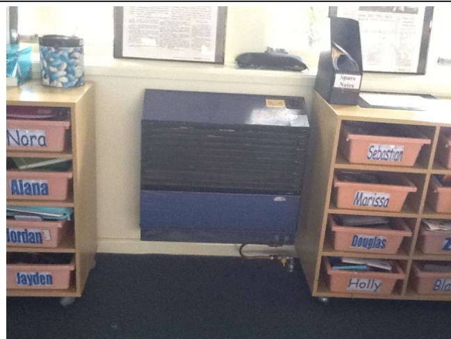
Photo No: J128920-003-Photo033 Result: Asbestos - Presumed Positive Building/Level: Building A-Ground Level Room/Location: R0010-North Feature/Material: Heater-Insulation
