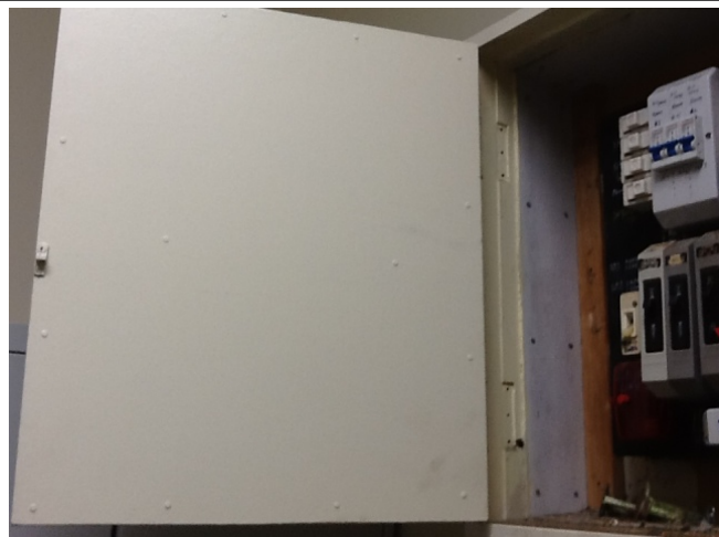
Photo No: J128920-003-Photo018 Result: Asbestos - Previously Sampled Positive Building/Level: Building A-Ground Level Room/Location: R0008-West Feature/Material: Electrical - Switch Board-Fibre Cement Sheetting
