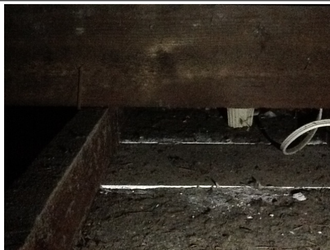
Photo No: J128920-003-Photo022 Result: Lead (Dust) - Positive Building/Level: Building A-Ground Level Room/Location: Ceiling Space-West Feature/Material: On Top of Ceiling-Dust - Lead
