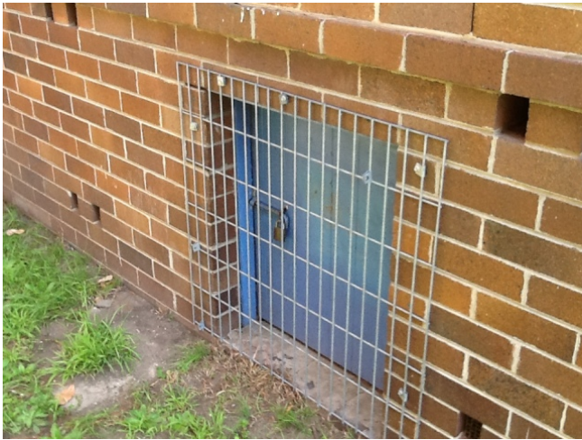
Photo No: J128920-003-Photo042 Result: Asbestos - Presumed Positive Building/Level: Building A-Sub-Floor Room/Location: Exterior-Throughout Feature/Material: Packer-Fibre Cement Sheetting
