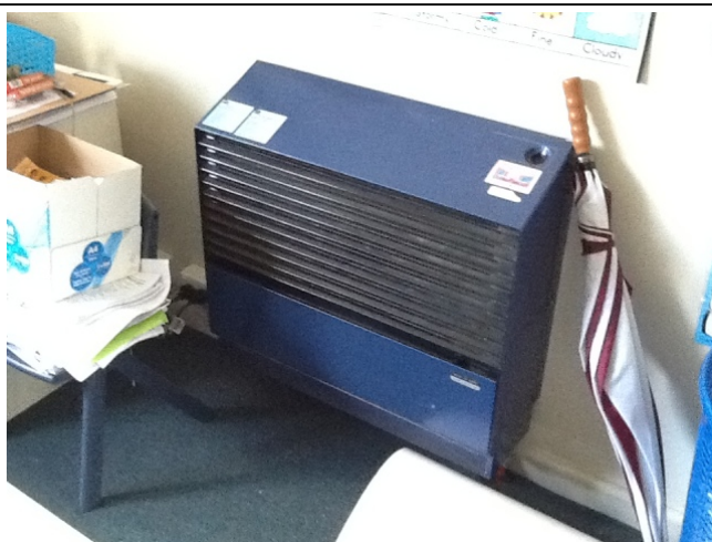
Photo No: J128920-003-Photo011 Result: Asbestos - Presumed Positive Building/Level: Building A-Ground Level Room/Location: R0005-North Feature/Material: Heater-Insulation
