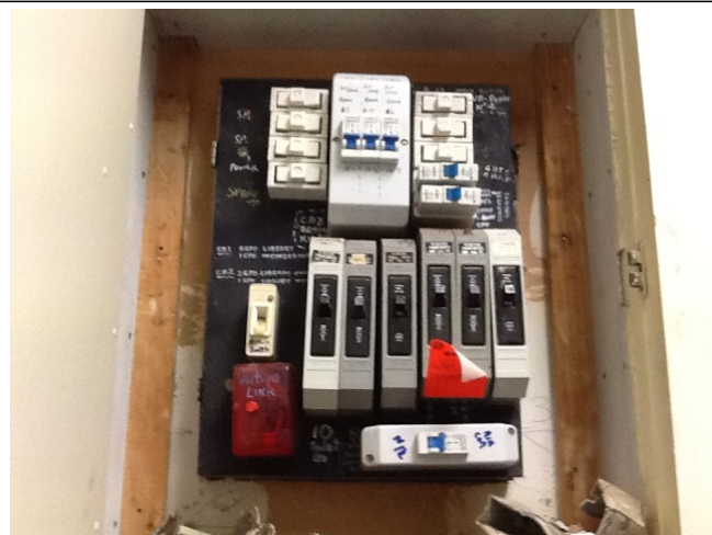
Photo No: J128920-003-Photo017 Result: Asbestos - Presumed Positive Building/Level: Building A-Ground Level Room/Location: R0008-West Feature/Material: Electrical - Switch Board-Compressed Bituminous Electrical Panel
