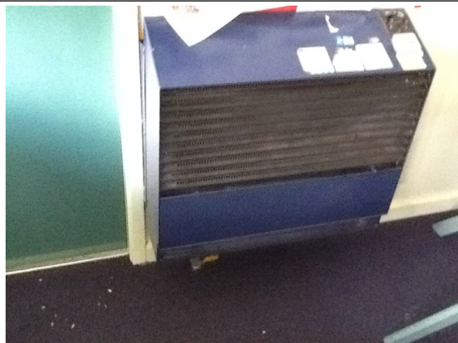
Photo No: J128920-003-Photo014 Result: Asbestos - Presumed Positive Building/Level: Building A-Ground Level Room/Location: R0006-North Feature/Material: Heater-Insulation
