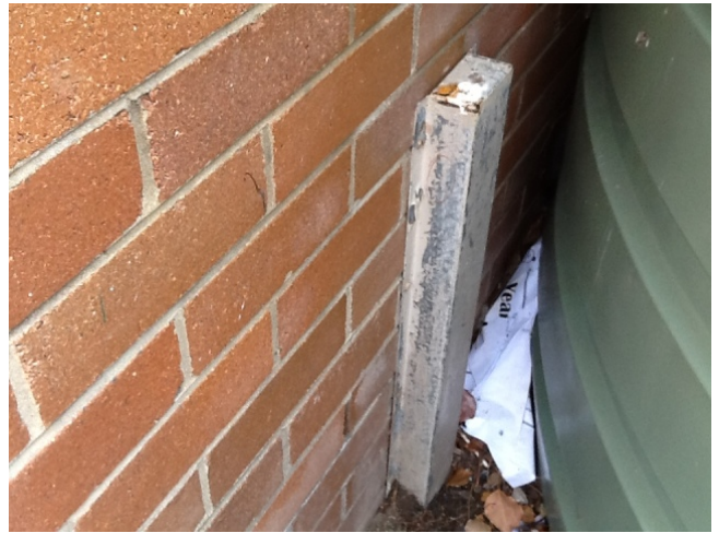
Photo No: J128920-003-Photo049 Result: Lead (Paint) - Positive Building/Level: Building B-Ground Level Room/Location: Exterior-South & East Feature/Material: Metal Work-Paint System/s
